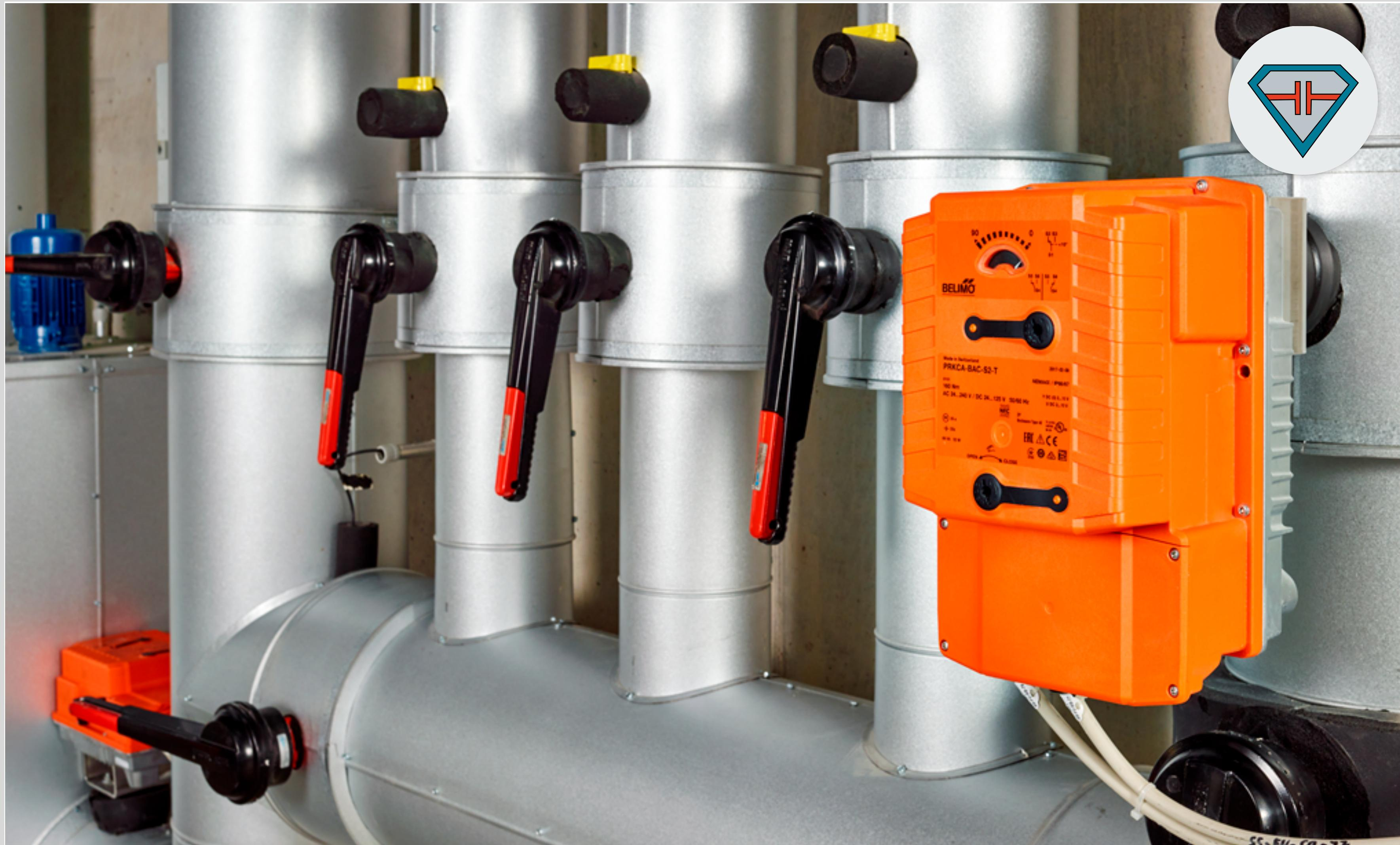
Actuator types with BACnet and SuperCap emergency control function:
